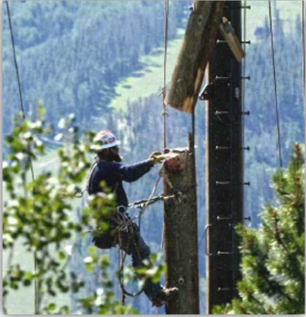
Linemen working on a distribution pole
