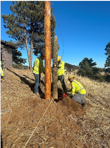
Linemen replacing a distribution pole
