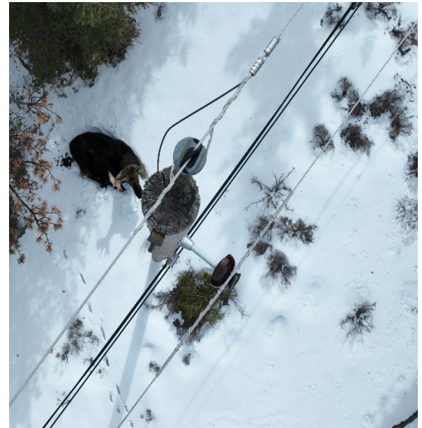
Overhead Pole Inspection
